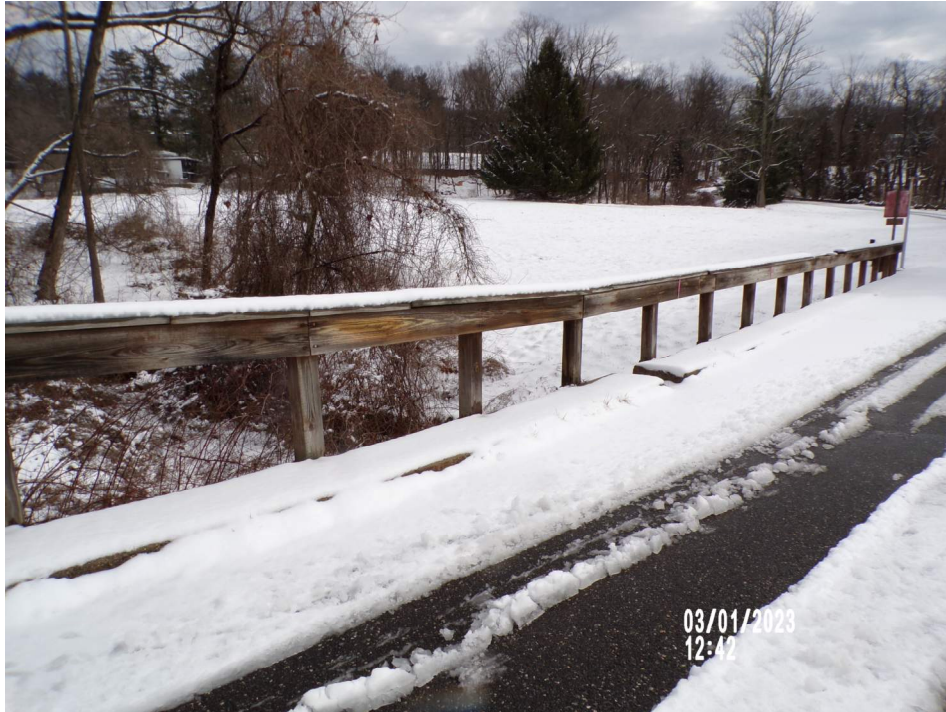
Photograph 3. Bridge Rail/Approach Rail, North Side
