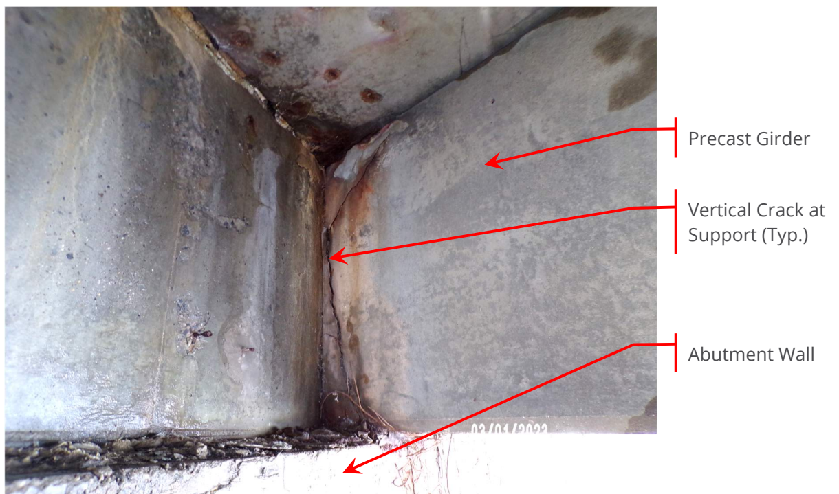
Photograph 14. Underside of Bridge
