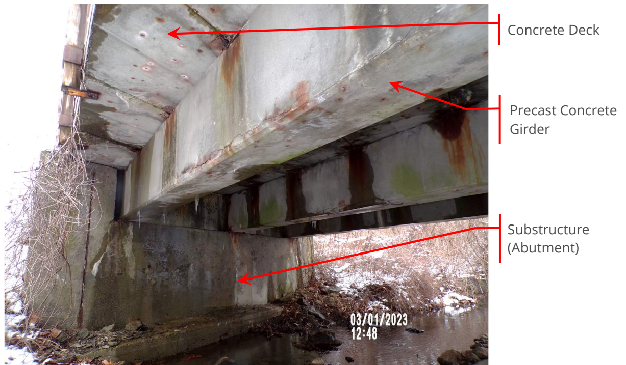
Photograph 7. Underside of Bridge
