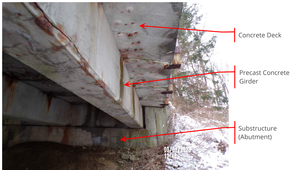
Photograph 8. Underside of Bridge
