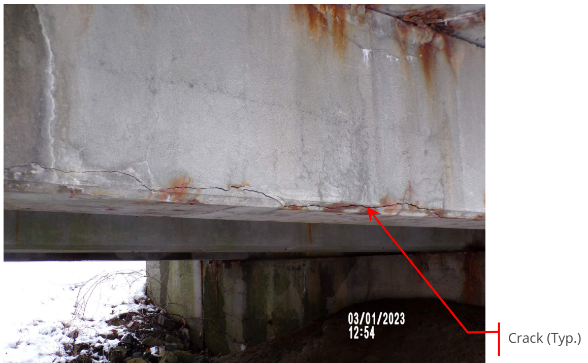
Photograph 10. Horizontal Crack Along Bottom of Precast Girder, Underside of Bridge
