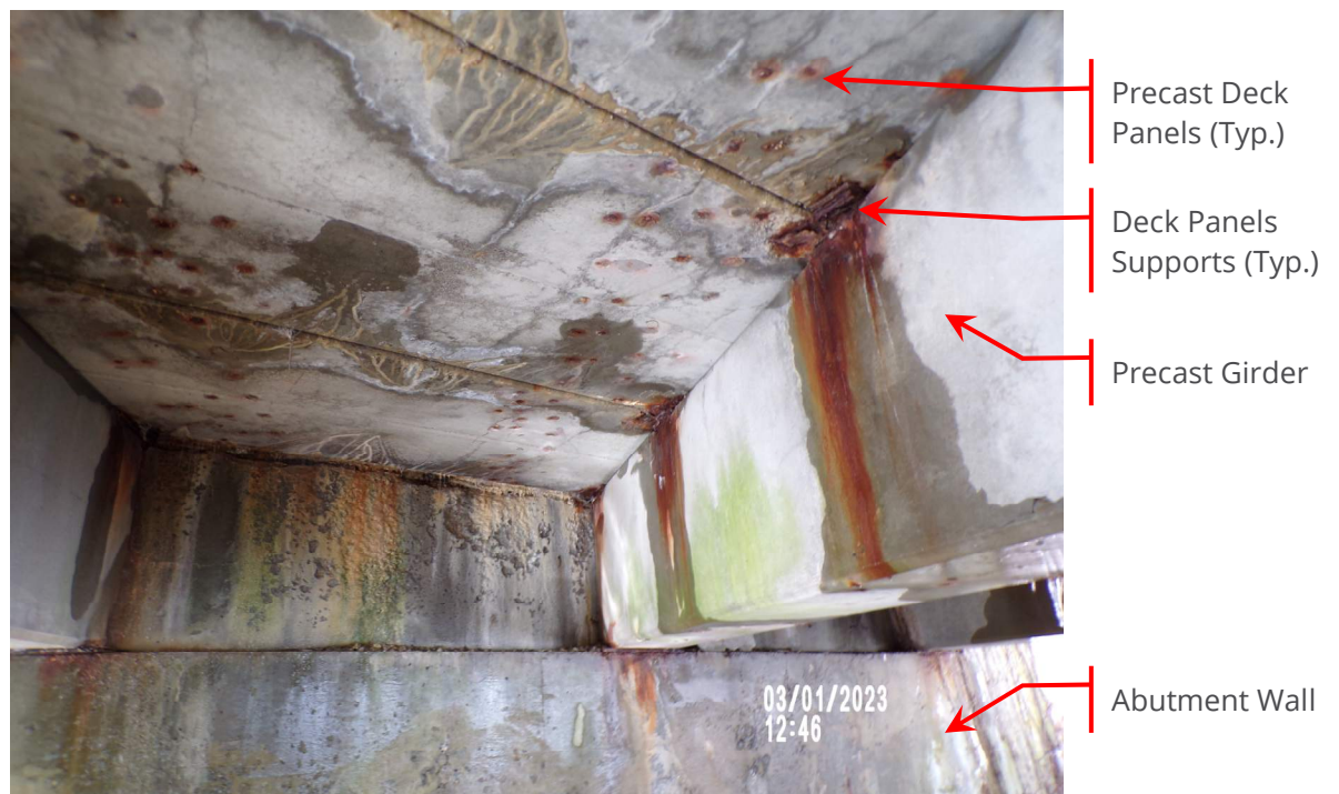
Photograph 12. Underside of Bridge
