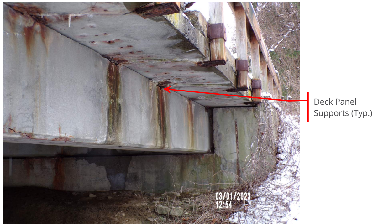
Photograph 11. Spalls and Signs of Corrosions, Underside of Bridge
