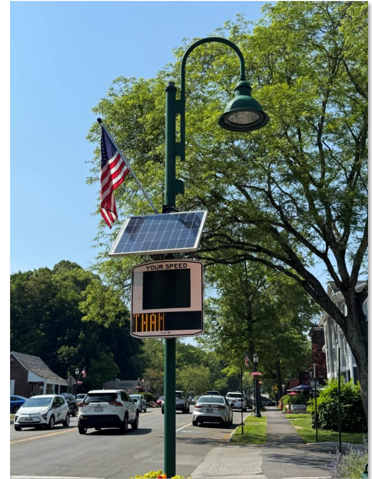
Solar-powered speedometer on Pleasantville Road
